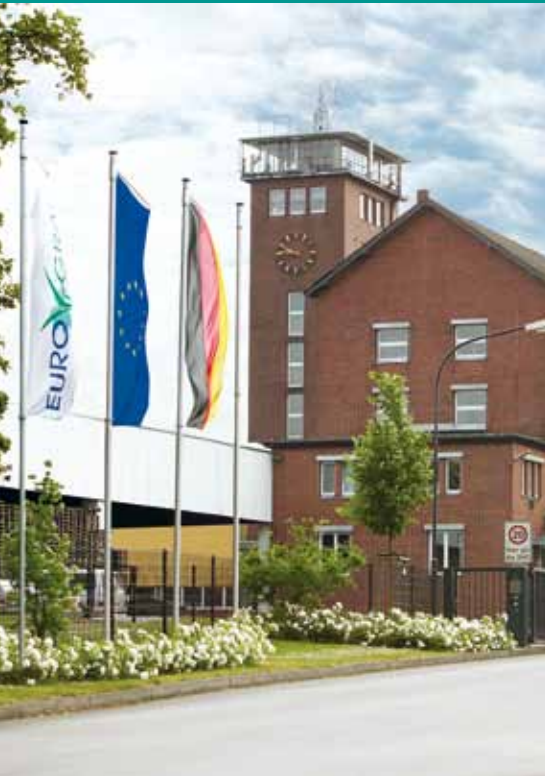
▲ DSV Headquarters Lippstadt, Germany
